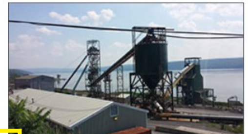
Surface plant facilities of the Cayuga Mine in 2013.
